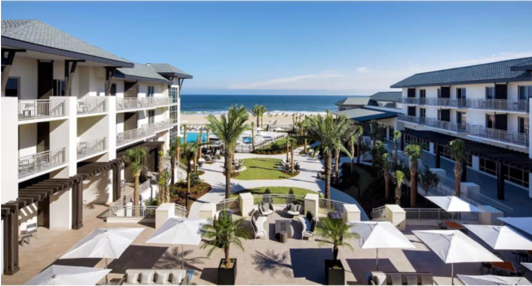
The resort's expansion includes the addition of a newly-constructed wing comprising 42 suites, amplification of event spaces and extension of the oceanfront pool deck. (Key International)
